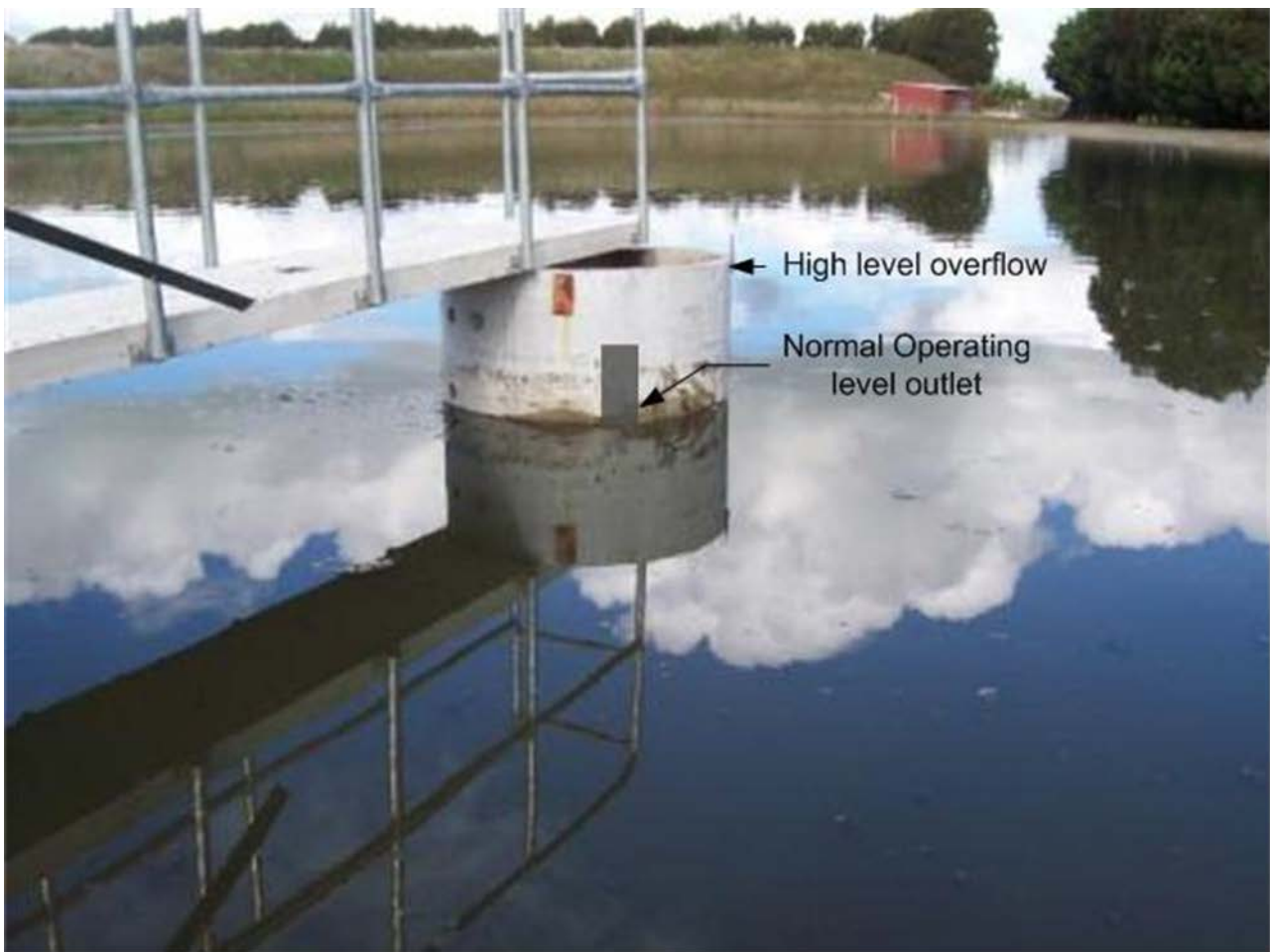
Figure 2-3 Outlet structure - allowing fixed outlet flows until pond is full
