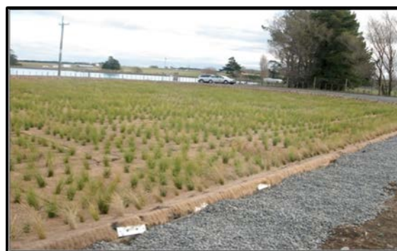
Figure 3-24 Anaerobic Pond Cover
