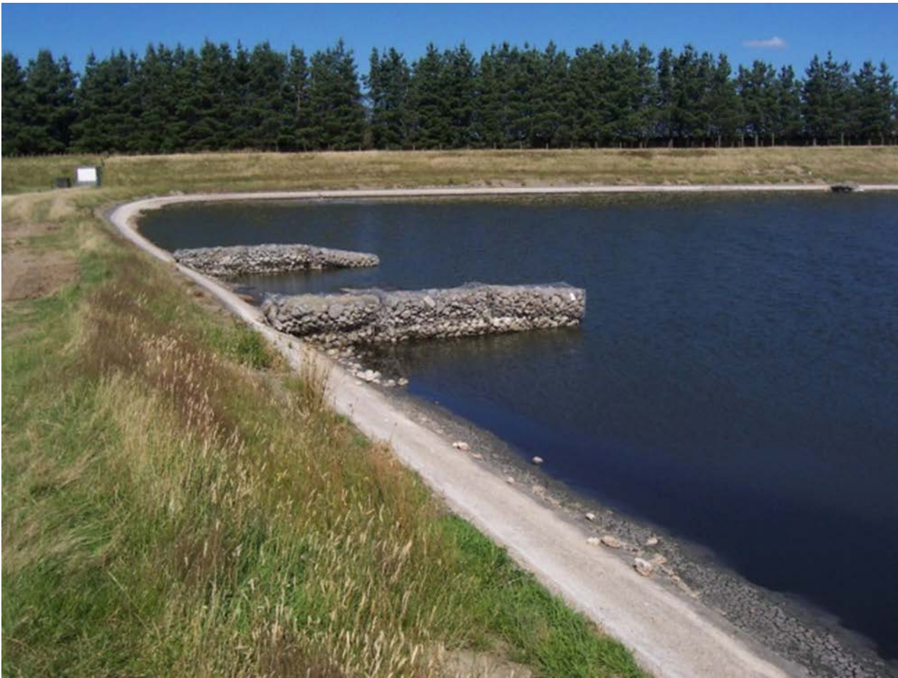
Figure 2-4 Outlet baffling using gabion baskets - outlet is between two stub baffles
