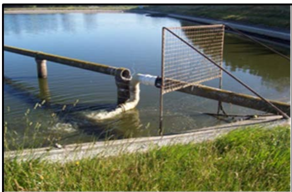
Figure 3-5 Jetting Inlet Upgrade
