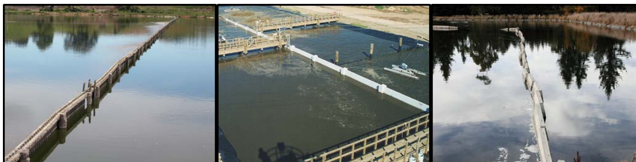
Figure 3-9 Old Fibre Cement Wall
