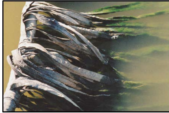
Figure 3-22 Inadequate Media Type B
