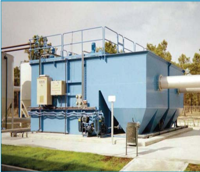
Figure 3-28 Actiflo Reactors
