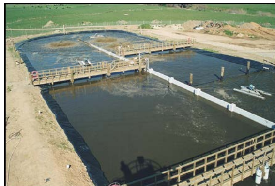
Figure 3-26 ... to an Activated Sludge Process
